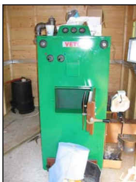
Fig 1: The Woodchip Boiler
