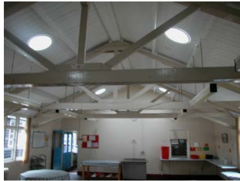
Fig 4: The Effect of the Sun-Pipes Inside the Building.
