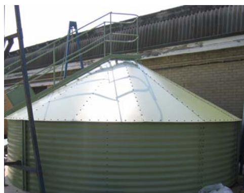
Fig 2: Chip Blower and Silo
